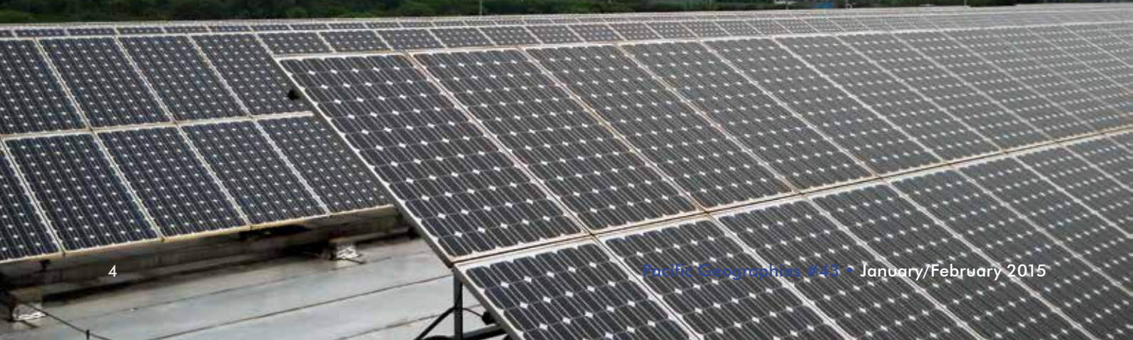
Figure 1: PV Panels in North China
