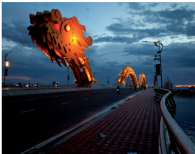
The Dragon Bridge: an essential part of Da Nang's urban identity
