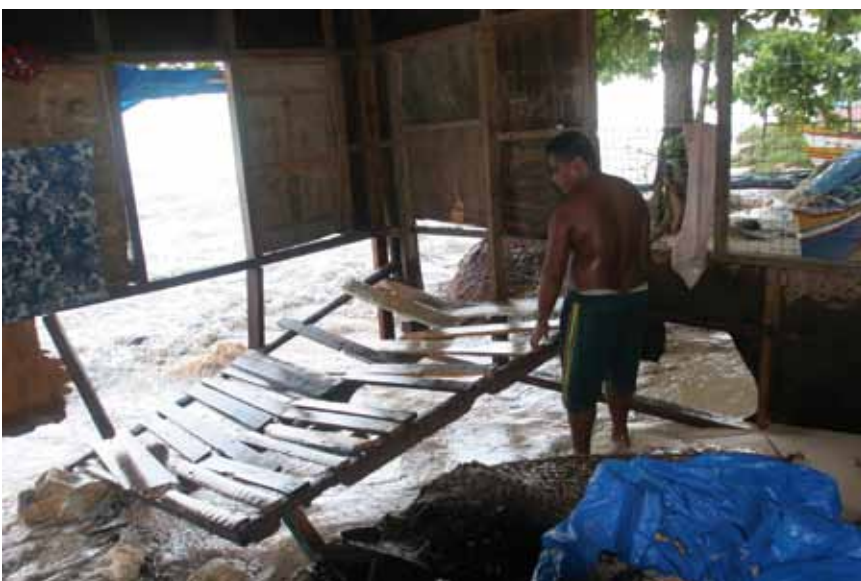
Waves from the ‘King Tide’ cause destruction inside the house, Tarawa Island, Kiribati
