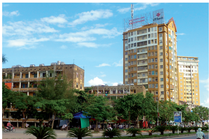
Quang Trung Zone C with the new TECCO Towers, for which residential building C1 was demolished in 2004
