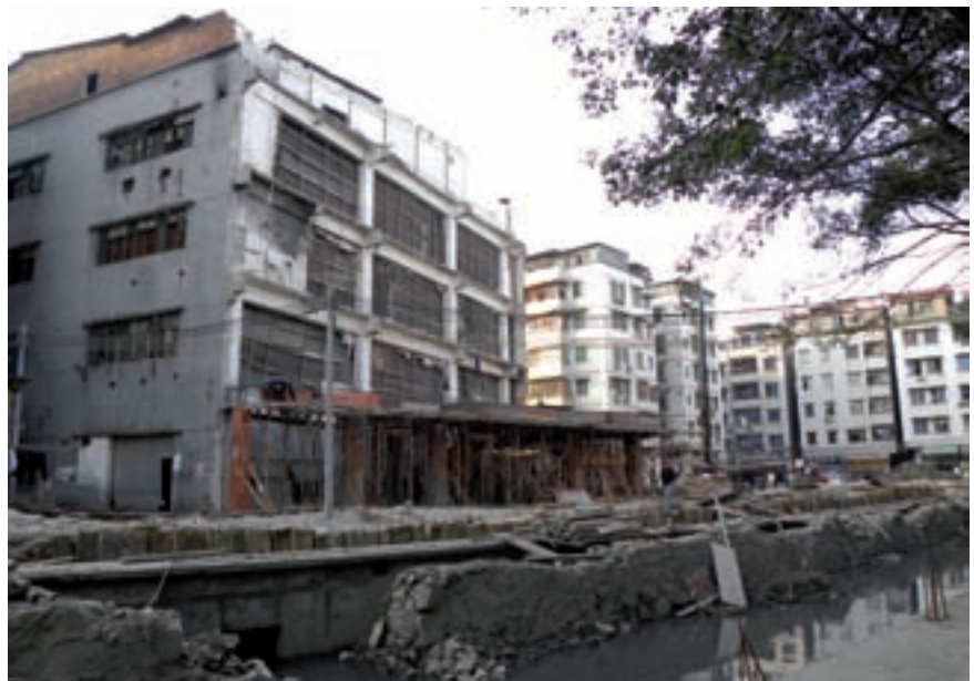
Demolition activities and upgrading along a canal
